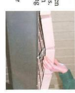
Step 3. Place cleat off the edge of the dock, next place (2) 1/4" x 3" hex head bolt & washers through cleat as shown Install cleat clip under decking and loosley hand tighten with a 1/4" flange nut.
